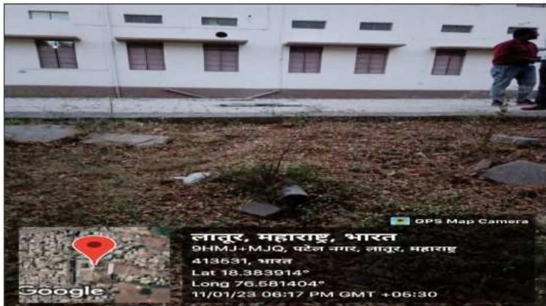
Drainage system for liquid waste disposal
