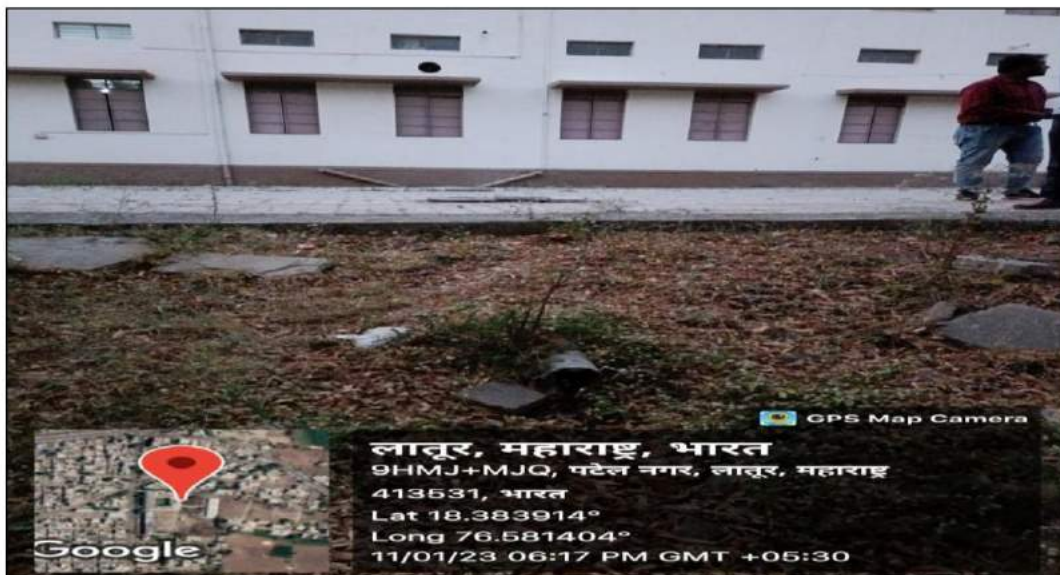
Drainage system for liquid waste disposal
