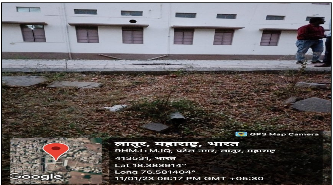
Drainage system for liquid waste disposal
