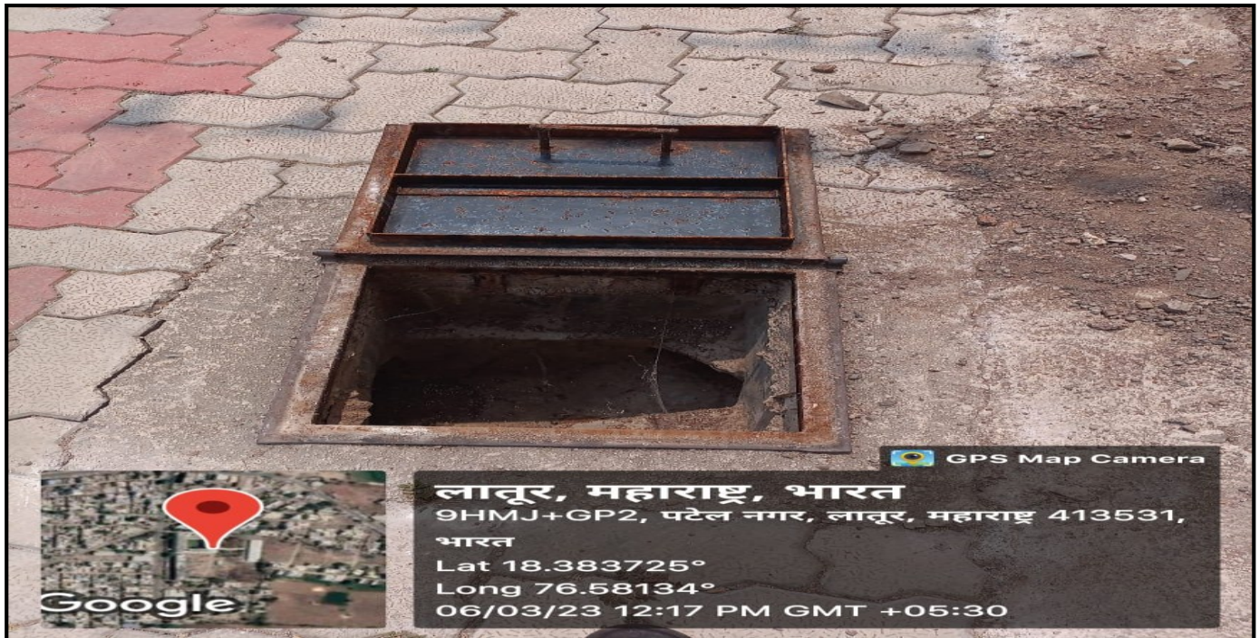
Liquid waste disposal soak pit
