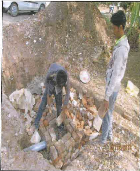
Construction of rain water harvesting pits
