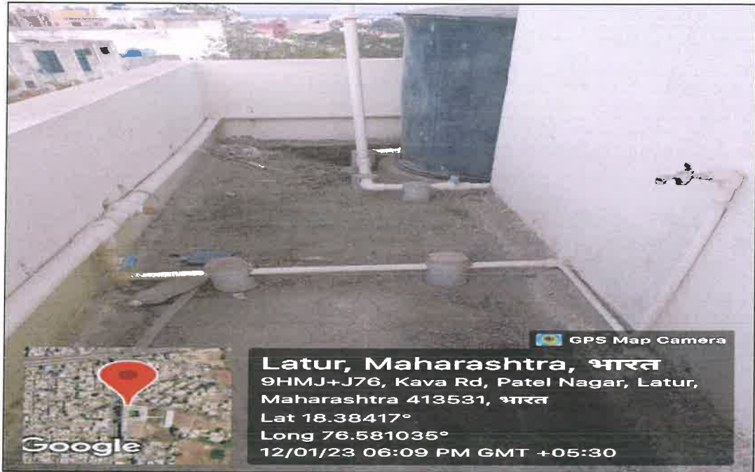
Wastewater treatment and reuse
